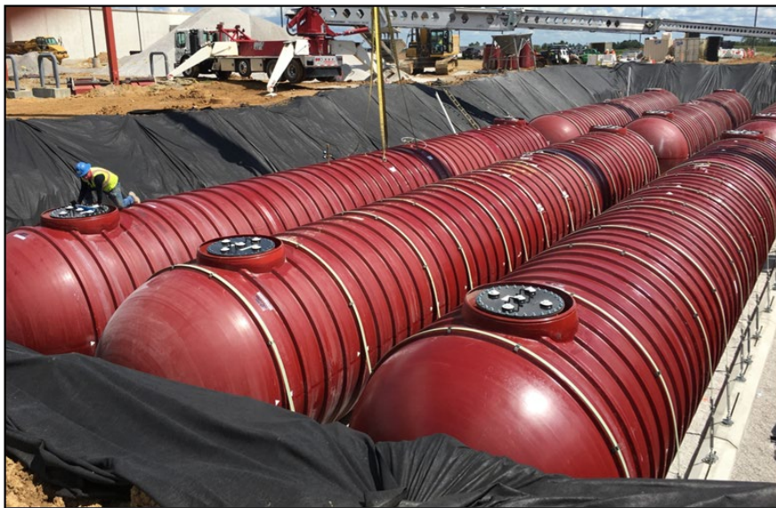
Photo 12: Underground Storage Tank Installation
