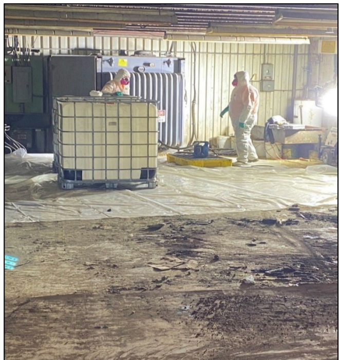
Photo 9: Kentucky Processing Prep Plant remediation
