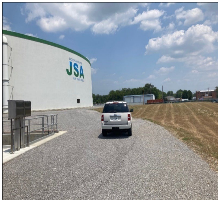
Photo 6: Paducah McCracken County, Joint Sewer Agency Tank
