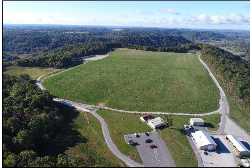
Photo 11: Maxey Flats, Post-Capping
